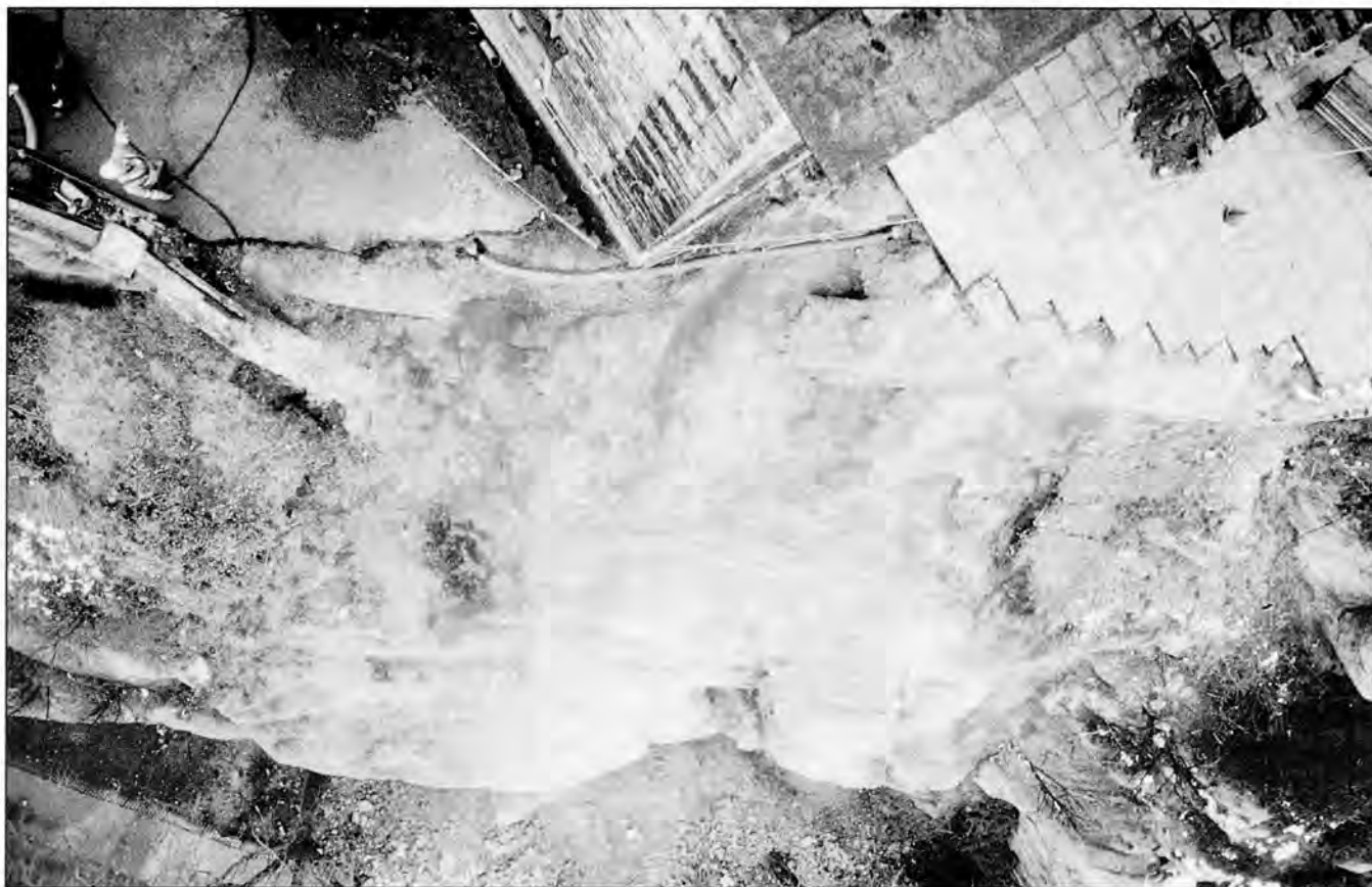
The landslide site seen from almost vertically above, after the loose debris had been cleared off. The straight line of the Norman wall is clearly exposed, as very little of it had fallen away; the gap in it dates almost entirely from about 1680, when space was created for the mansion foundations.
