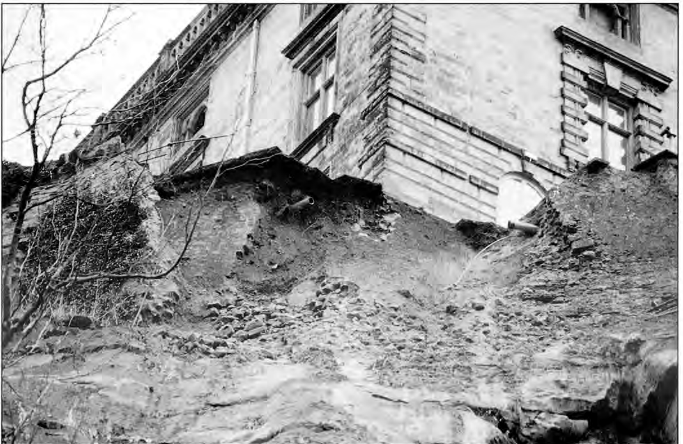
Closer view of the slide scar, with the masonry of the Norman wall visible beneath the overhanging terrace paving; undisturbed sandstone is exposed at the foot of the picture.
